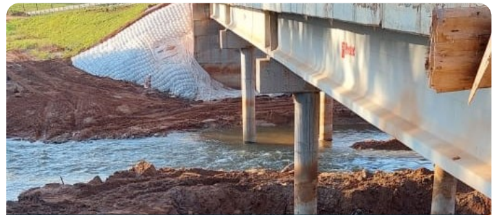
Articulated Block protecting the abutment and the piers — Gasory Stream Bridge, Paraguay
