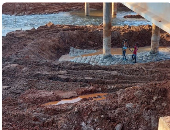
Bridge pier protection — built with the same system
