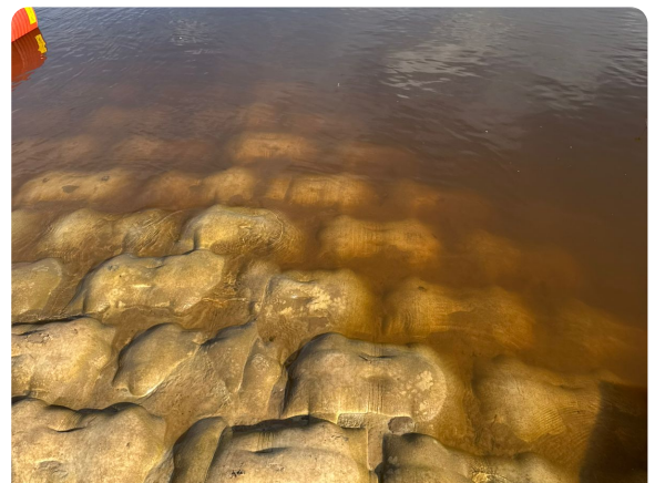
Mattress filled underwater, in service
