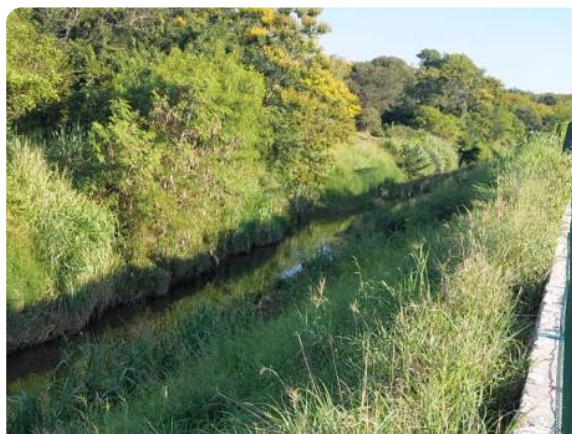
The same reach, fully revegetated
