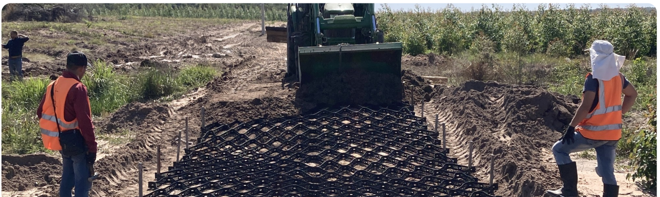
Forestry road reinforced with 100 mm StrataWeb® within the plantation: the cell is filled with the material from the site itself — Concepción
