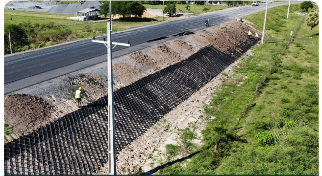
57,000 m 2 of slope lined with StrataWeb® — Alberdi approaches
