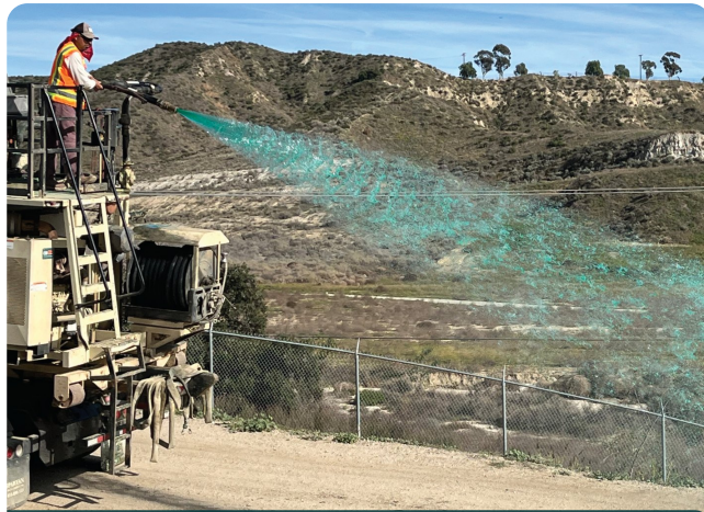
Application of DustRX Hydro — the green marks the coverage
