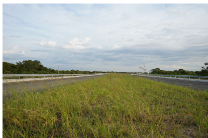
Dense turf on the embankment — the finished result
