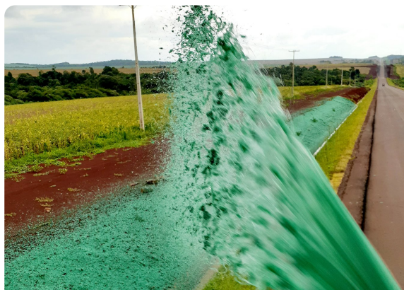
Hydraulic mulch applied with the cannon — the green colour marks the coverage
