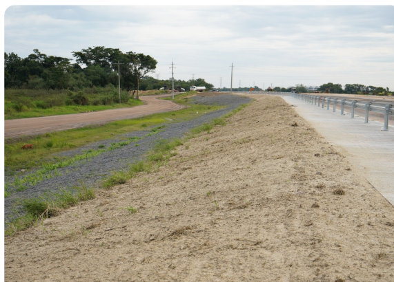
Hydraulic mulch freshly applied — protection from day one
