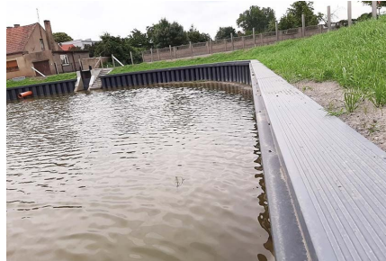
Urban channel with a pedestrian promenade over the capping
