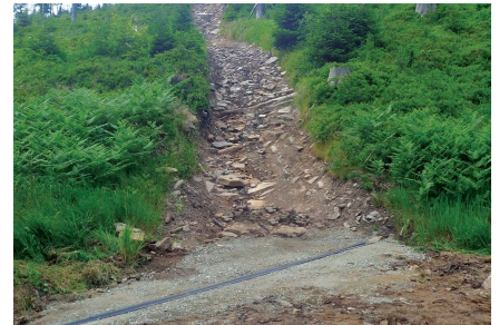
Road drainage: a lined channel that does not erode
