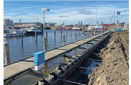
Wharves and moorings: no corrosion at the waterline
