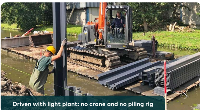
Excavation shoring in an urban area
