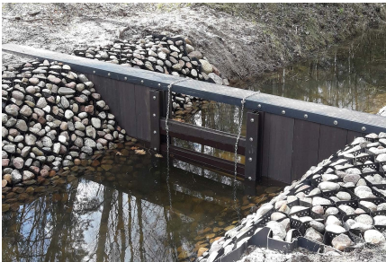
Hydraulic works: spillways, gates and weirs
