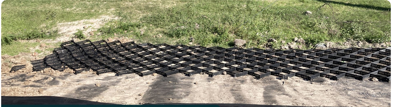
Soil reinforcement with Strata geosynthetics — road project in Paraguay
