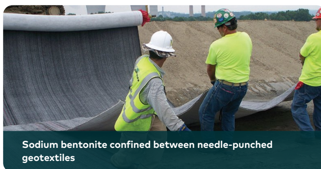
It is rolled out, overlapped and covered: no welding
