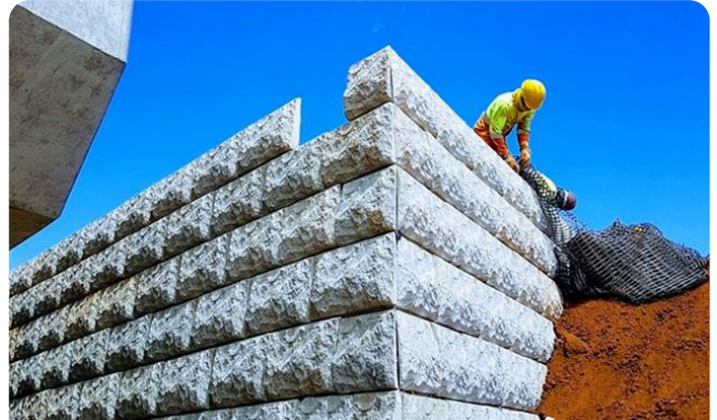
The stacked module and the geogrid that anchors it to the mass — a Lock+Load wall under construction
